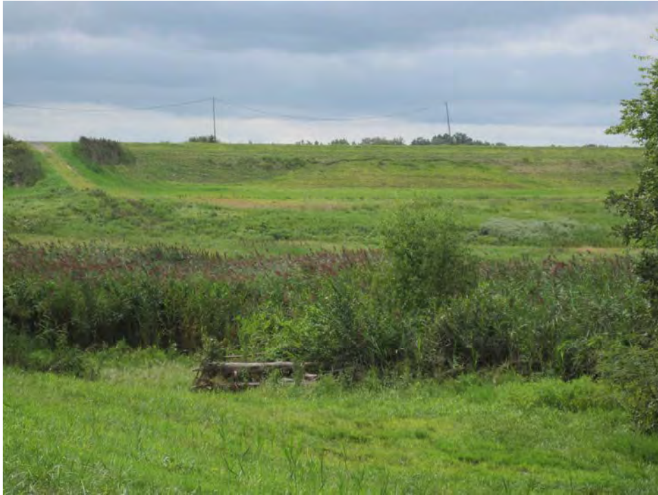
Figure I.1. Photo of 2015 surficial movement prior to repairs.
